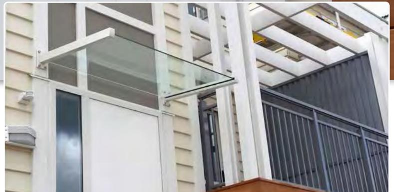
Edge® Canopy Awnings are designed and custom made in New Zealand using high quality aluminium extrusions and toughened glass infill.
